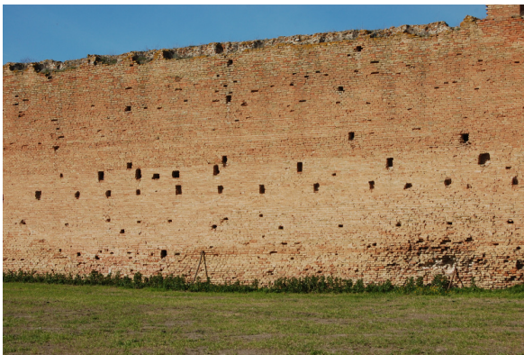
Fig. 2. Brick walls Angevin (XIII century)
